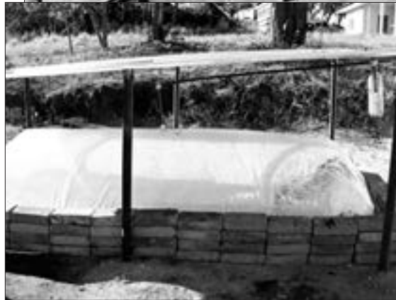
BioGas generator at Nicaragua
